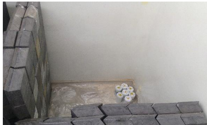
FIGURE 6: Waste storage area.
